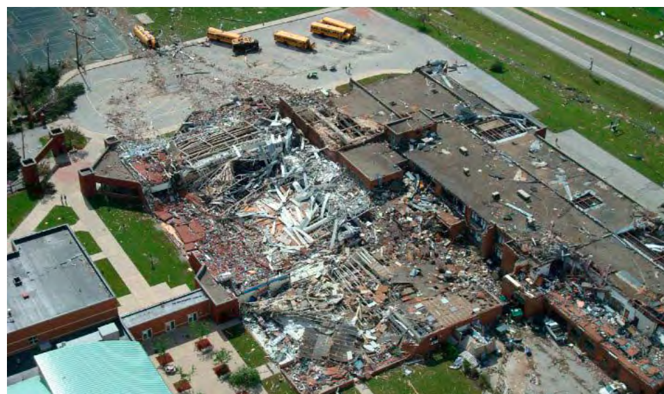
The destruction at Lake High School
